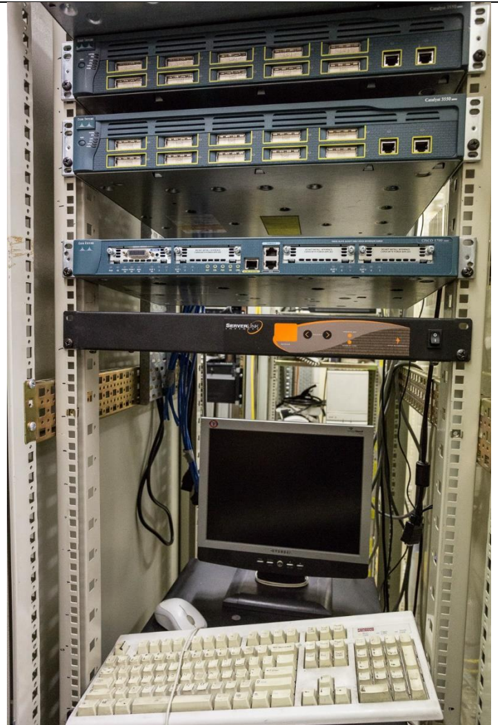
Suite 2A, Rack 3. Top of Suite 2 UPS rack, spare fibre switches and KVM.
