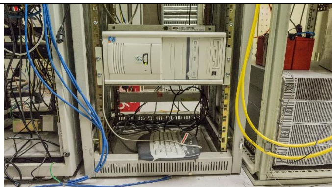
Suite 1A, Rack 3. Fog Server (Contains OS images for Training room PCs) Visible on right is 3KVA UPS with 3 extension batteries. On top is 2 additional batteries for the Security cameras.
