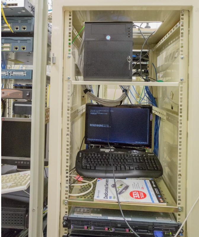
Suite 2A, Rack 4. Backup NAS (Network Attached Storage) & VMware host. The operating system for the NAS box is NAS4free BSD.
